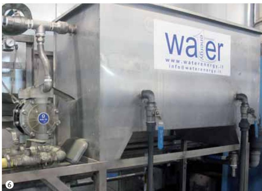
**Figure 6:** The separator for the removal of mineral oils from the pre-treatment tanks.
