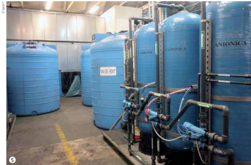
**Figure 5:** In the foreground, the two columns of the demineralisation system: one with cationic resins, the other with anionic resins.
