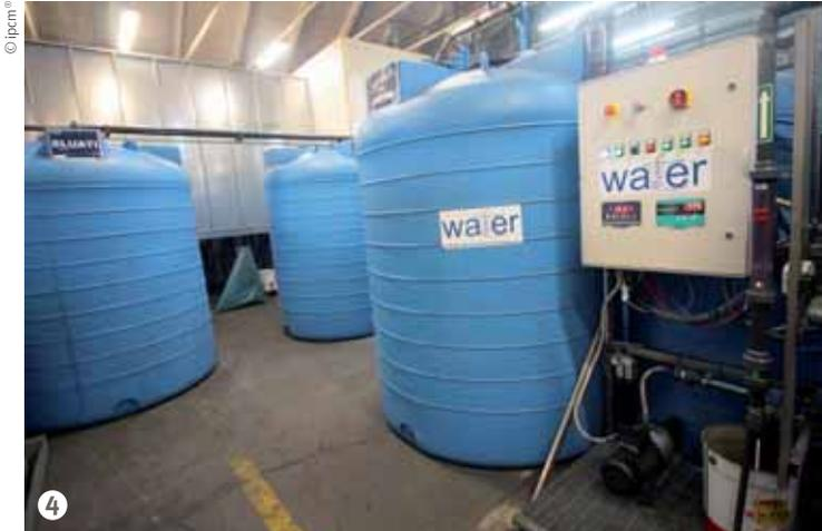
Figure 4: On the left, the non-hazardous eluate collection silo and, on the right, the control panel for the management of the water treatment system.
